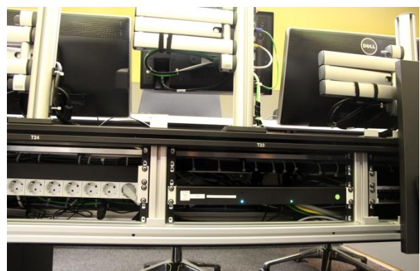
Workstation: back view (incl. CON Unit)
